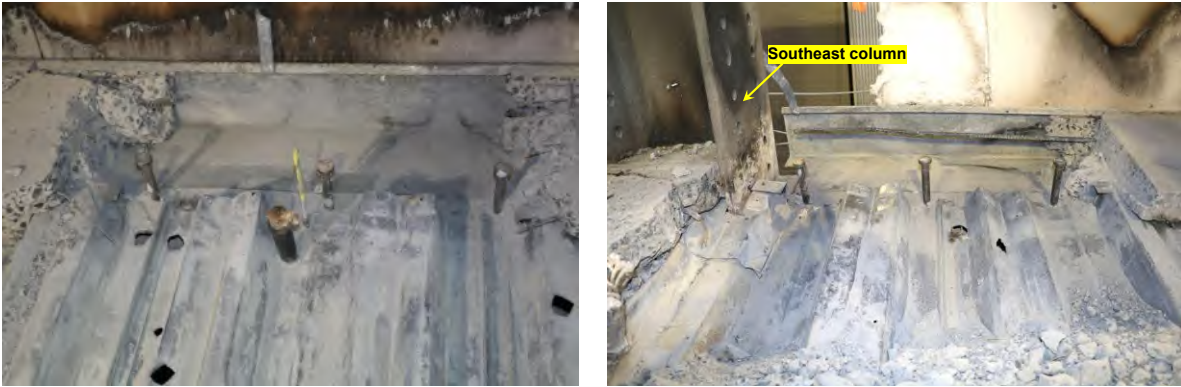
e f Fig. B-23. Post-test photographs of headed stud anchors in the test bay.
